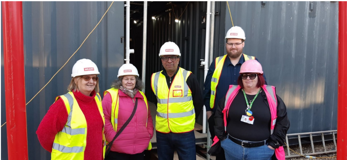
Members of the TFG on a site visit to the new modular housing development at Pencarrow Place, Fishermead
